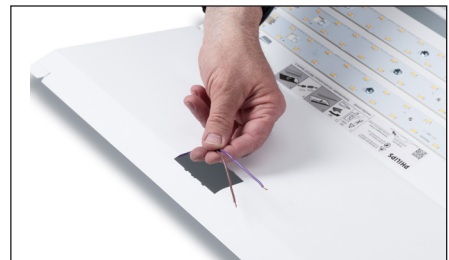
Step 3: Remove the two wires that were secured to the back of the plate.
